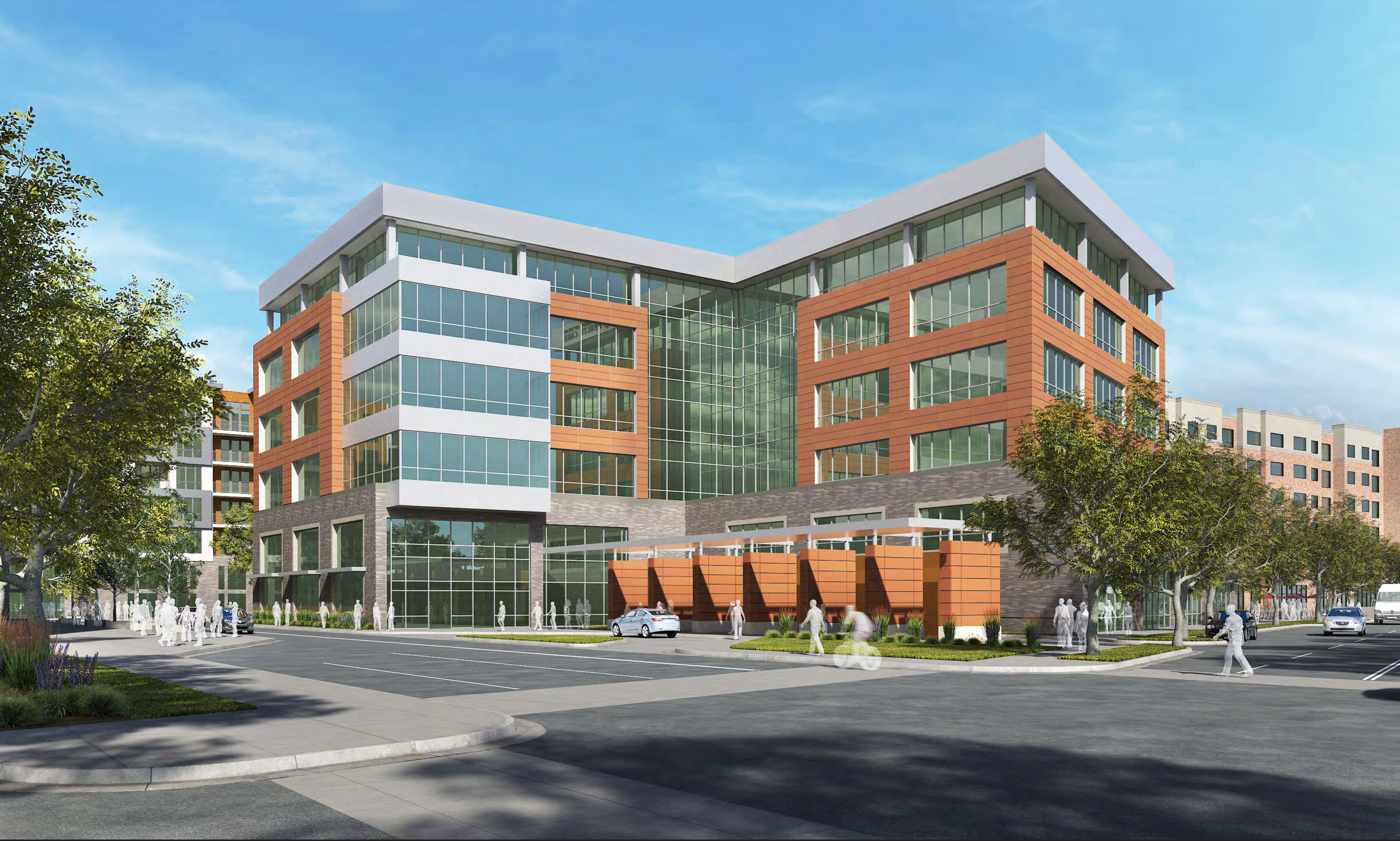
THE DIXON BUILDING NORTHWEST VIEW FROM WILMINGTON-HIGHLAND JUNCTION
